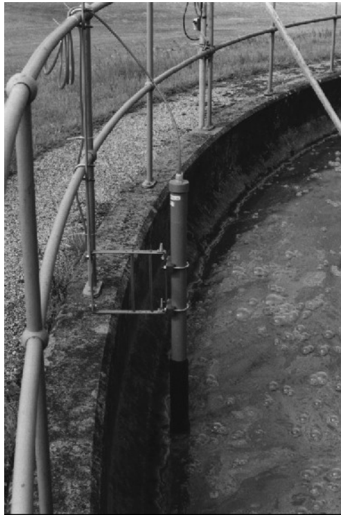
Figure 2 Typical TT2000 Installation
